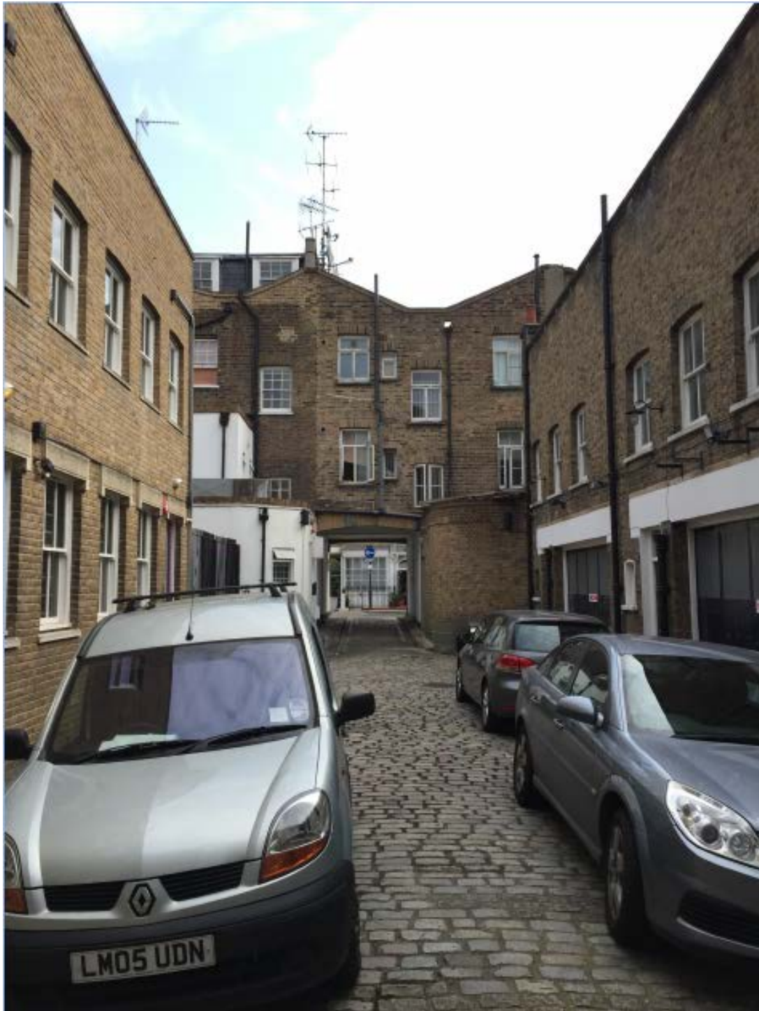
View looking up Rainsford Street toward Sale Place (site on right).
