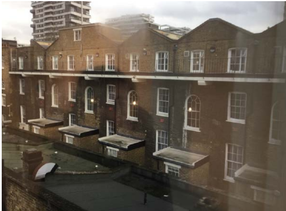
View of roofs of application site with Wilson House student halls of residents behind.
